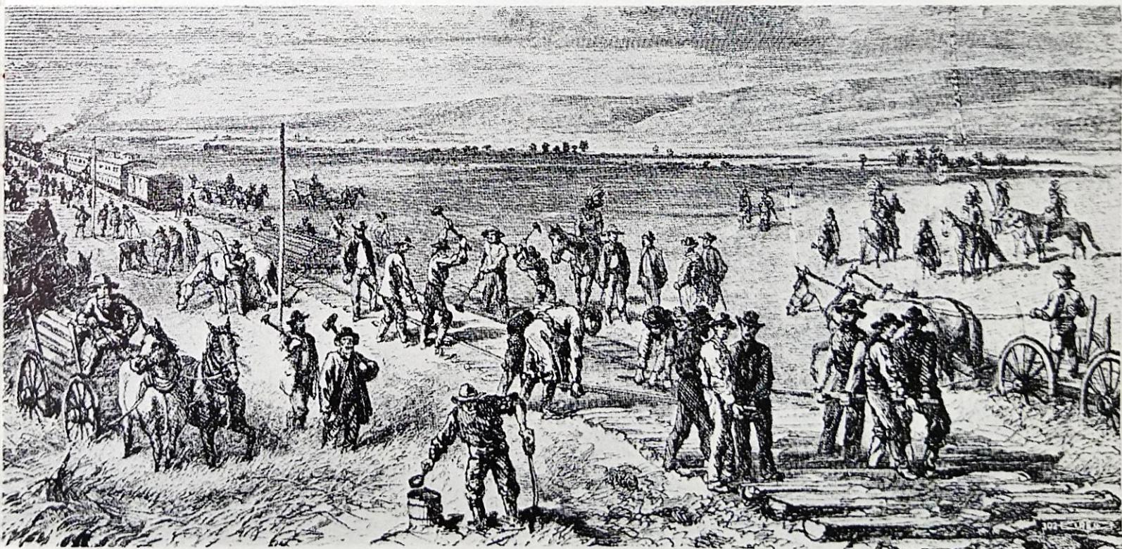
A typical scene of early railroad construction across the prairies.
